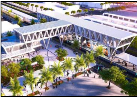
Next High Performance Rail system to open in North America: All Aboard Florida, Miami-West Palm Beach-Orlando. Drawing of the Ft.Lauderdale station, T-shaped with distinctive V-columns and glassed-in spaces, limited to two tracks centre platform. Story on Page 4. (Rendering: AAF)
