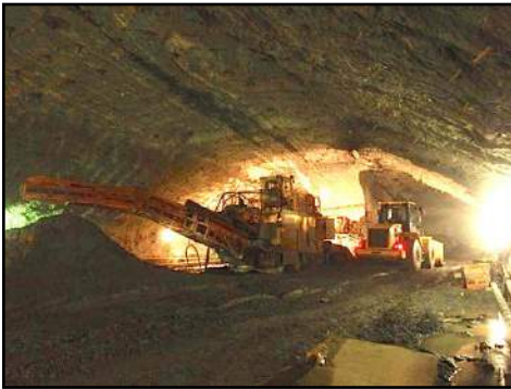
Digging out underground LRT station in Ottawa. Photo: Rideau Transit Group.
